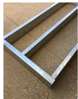
Joists fixed to "boxed-bearer".
