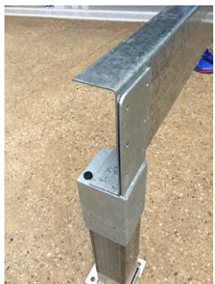
"D" bearer section ready to be fixed to "C" with "J" Tek's.
