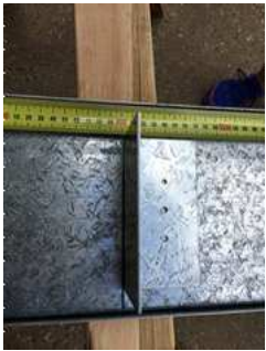
Fix brackets about mid height of bearer.
