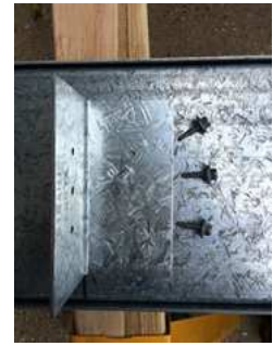
"G" bracket ready to be fixed to "E" with "K" Tek's.
