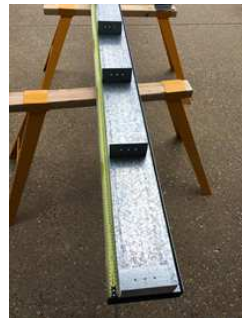
"G" brackets fixed to "E" bearer section. Can be done prior to assembly on stumps, or after.
