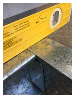
Tops of joists finish smooth, flush & level with tops of bearers.
