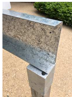
"G" brackets fixed to "E" bearer section. Can be done prior to assembly on stumps, or after.
