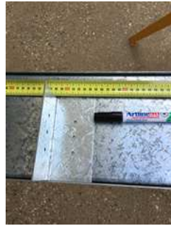
HINT. Use a joist bracket, as a square (held against the bearer's edge) to draw a vertical line.
